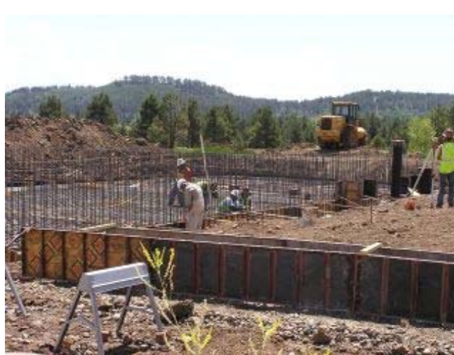
Lower slab foundation preparation
