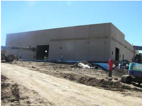
Exterior of the new Hatcher WTP
