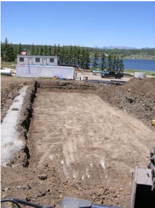
Lower slab excavation
