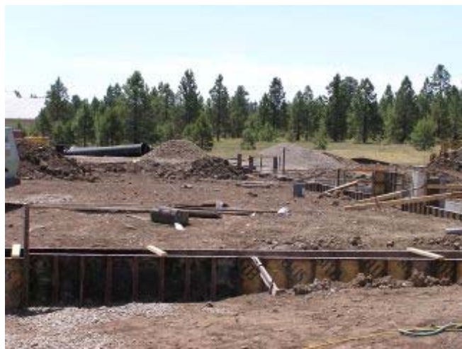
Preparation of upper slab
