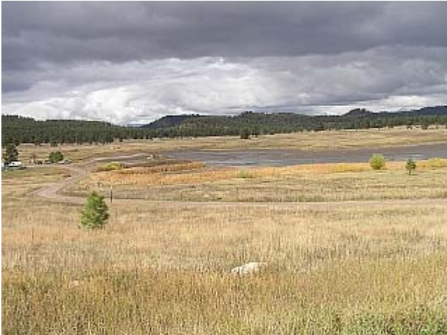
Looking west down the length of the dam
