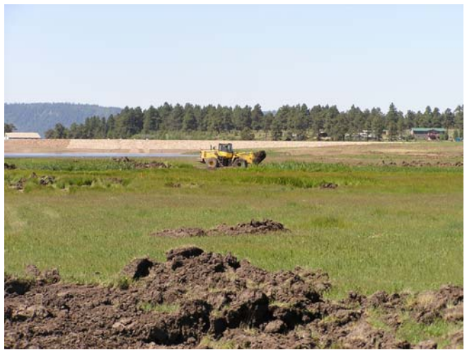
Placing 27 acres of wetlands soils, a bucket at a time
