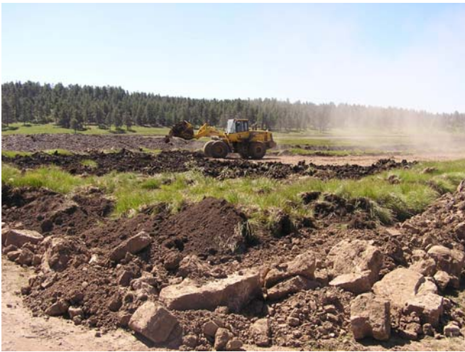
Wetlands soils, in place and ready for planting
